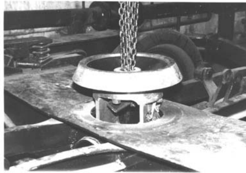
Figure 3 – Moment from the assembly of the force transducer in the king-pin bearing beam
