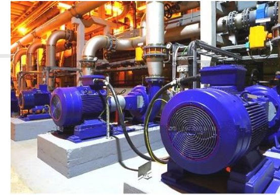
Induction motors - the driving force of the pumping station
