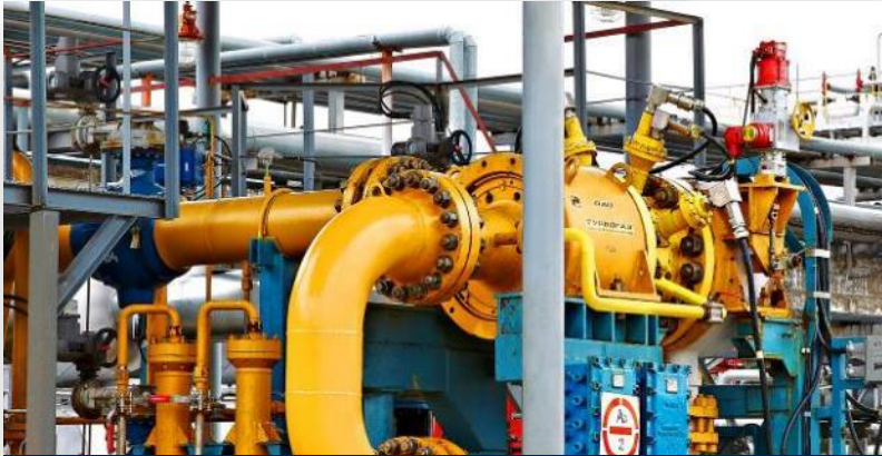
Expander-compressors for preparation and treatment of natural and associated petroleum gas
